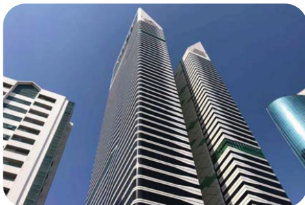
Nassima Tower, Dubai
