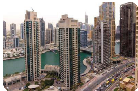
Trident Grand Residence at Dubai Marina, Dubai
