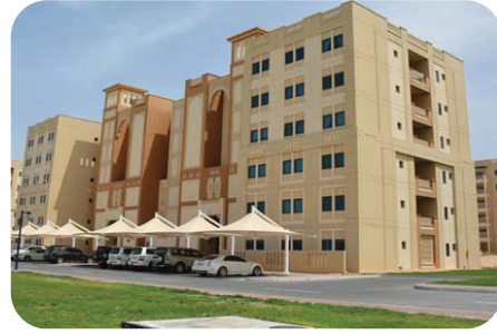
Adnoc Residential Complex at Khalidiya City, Abu Dhabi
