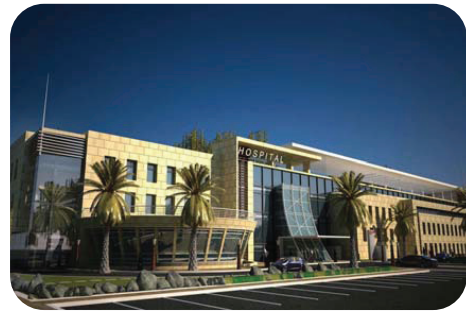
Dar Al Shifaa Hospital in Khalifa City, Abu Dhabi
