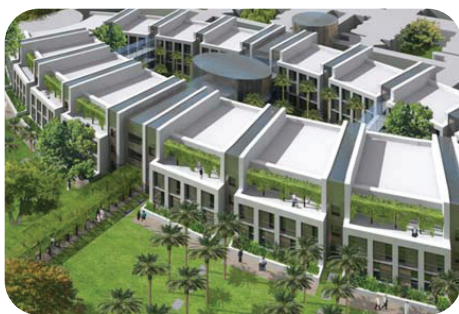
Al Wasl Maternity Hospital, Dubai
